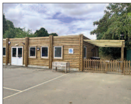
PURPOSE-BUILT: The Cabin at Gamlingay is now completed.
